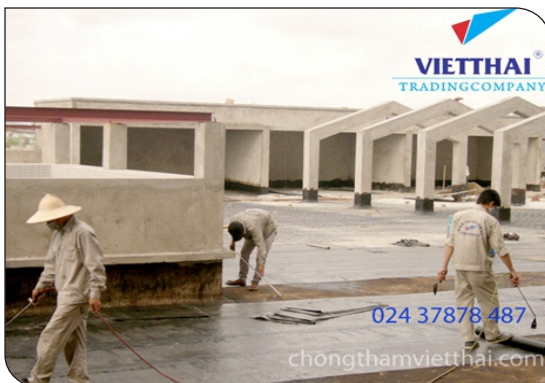
Construction of torched on membrane
